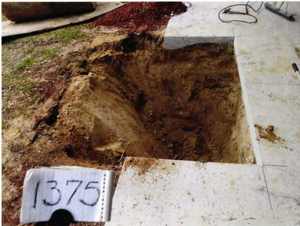
Picture 2: UST 1375Dove excavation.
